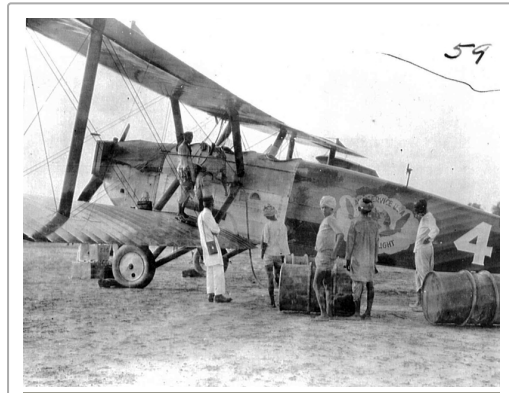
The New Orleans gets serviced in Allahabad, India. (342-FH-3B-8142-11878AS)
